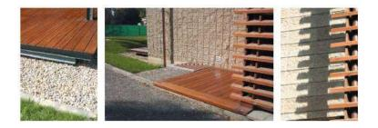
Figure 9. Timber floors and sun barriers in conjunction with masonry walls.
