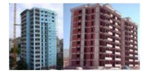
**Figure 1:** Polystyrene based foam used in insulating buildings for thermal effects on a clay brick facade wall on the left and before insulation and plastering on the right.
